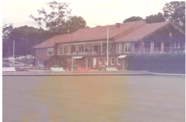
Work is complete
