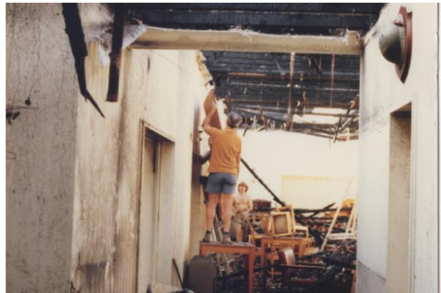
The clean up begins
